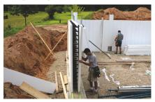
**VERTICAL ICFS** have all the energy efficiency, strength and building speed benefits of conventional ICF walls but go up faster and easier because fewer pieces are assembled on site.
